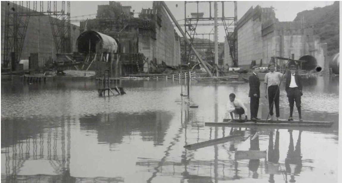
National Archives at College Park, Record Group 185g, Box 3, Vol. 6. Photo caption: "33-G3 Pedro Miguel Locks. Looking North from South End During Flood - December 4, 1910."
